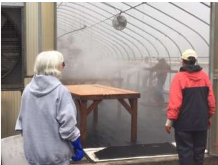
Power washing inside the greenhouse
