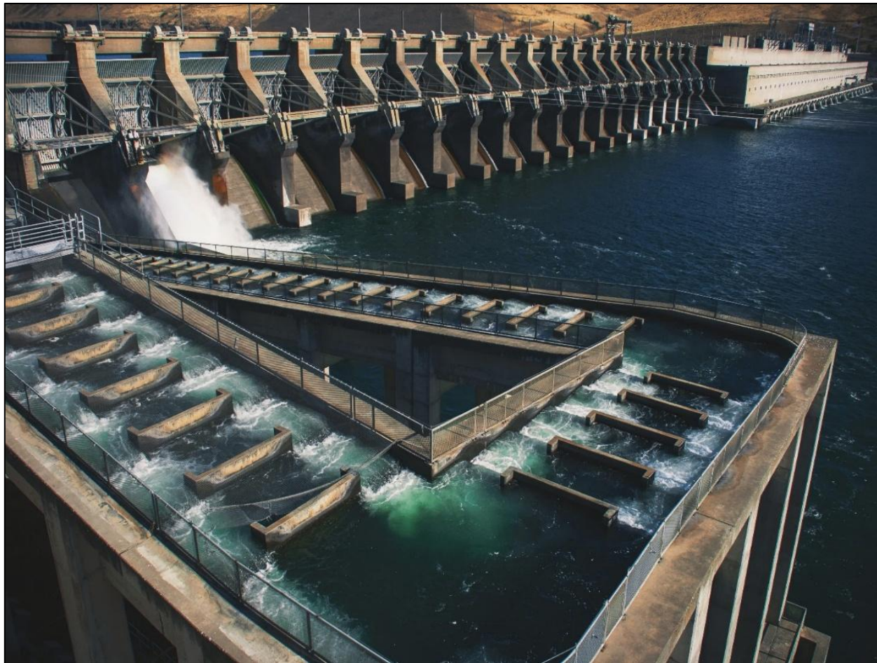
Figure 1. Fishways are designed to facilitate dam passage of returning upstream-swimming adults and downstream-swimming juveniles. To a degree, these structures work, but the collective negative effect of dams (and many other threats) reduces the quality of the overall environment for most anadromous species. One result of using such technological solutions is an optimism bias that pervades the SRIC and creates unrealistic expectations by the public and some elected or appointed officials about what level of salmon recovery, if any, will be achieved by the billions being spent. (Photo courtesy U.S. Army Corps of Engineers)
