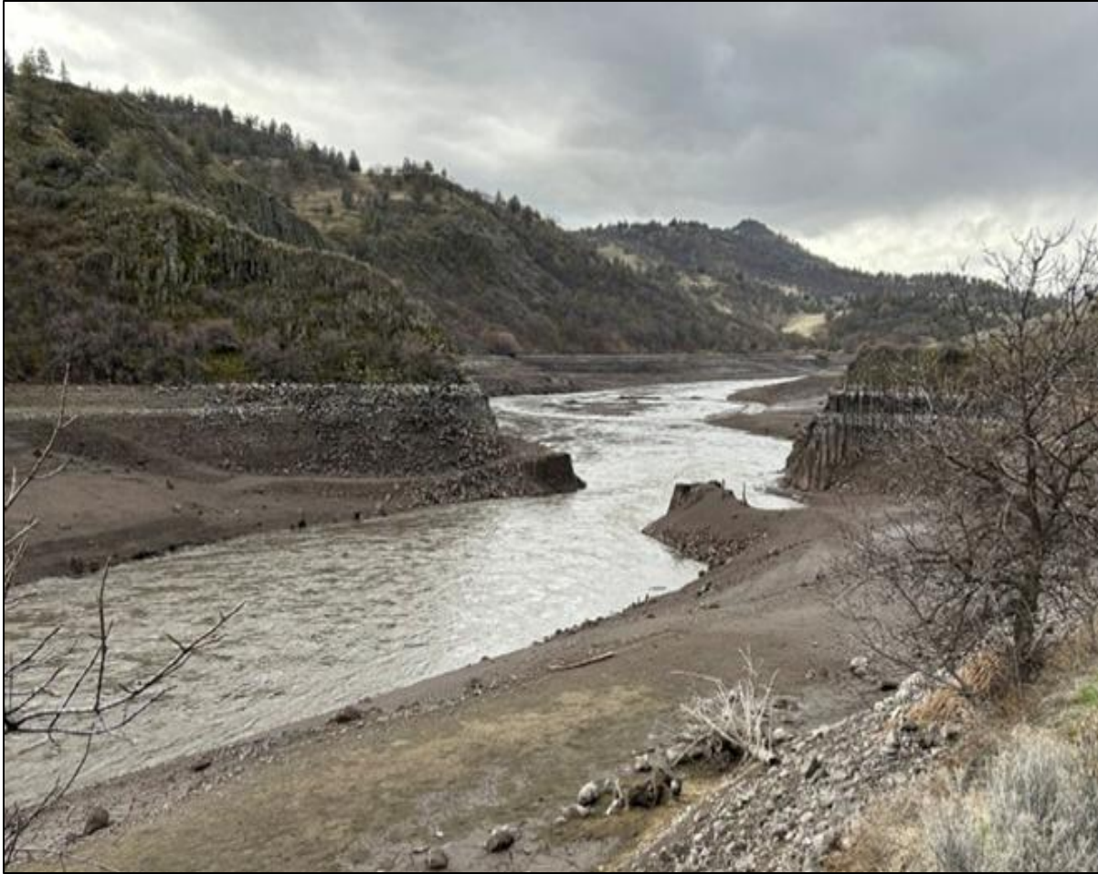
Figure 3. Four Klamath River dams near the California-Oregon border were recently removed after years of political controversy (the location of one dam is visible in the center of the photograph). The removal of these relatively large dams became politically viable when they were no longer profitable as electricity producers, supplied a relatively small number of farmers with irrigation water, and afforded minimal flood protection. (Photo courtesy U.S. Department of the Interior)
