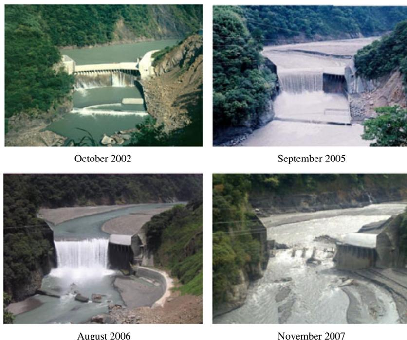
**Figure 2.** Sequence of photographs looking upstream at Barlin Dam and its failure in 2007. Note the exposure and extent of the reservoir sediment in 2005. The defense dam, which was critically damaged during Typhoon Aere in 2004, completely failed in 2006. (Photos courtesy of Taiwan Water Resources Agency, used with permission.)
